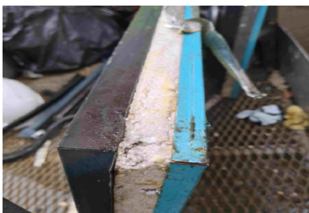
3.8.4 External Block Wall with facing Stone
