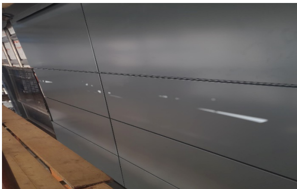
{Newly installed cladding image}
